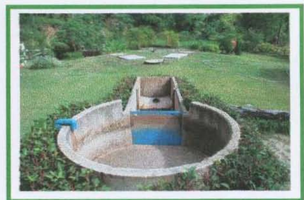
Figure 13 : Fixed Dome System (after Land Reclamation)
