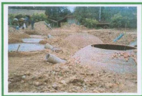
Figure 12 : Fixed Dome (Under Construction)
